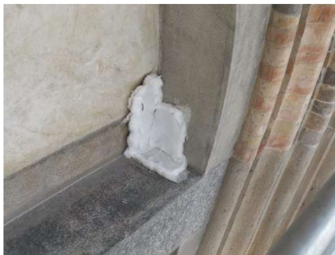
3 Cleaning with cellulose-based compress
