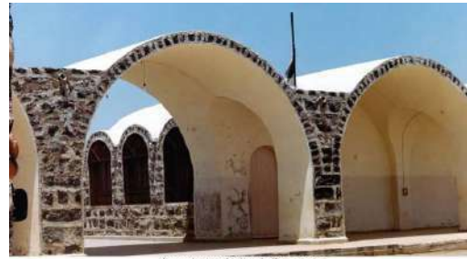
Archway and circulation area
