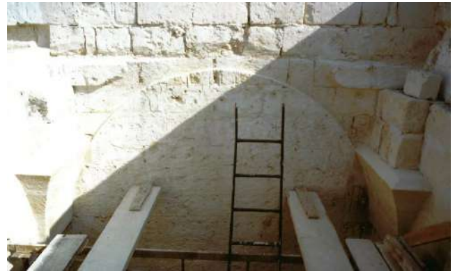
Photo 4: once the design is traced, a recess is made so that the blocks of the vault rest firmly on the wall.
