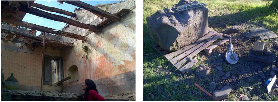
5 – type of existing and used materials: wooden beams, lime plaster, gray tuff from Campania.
