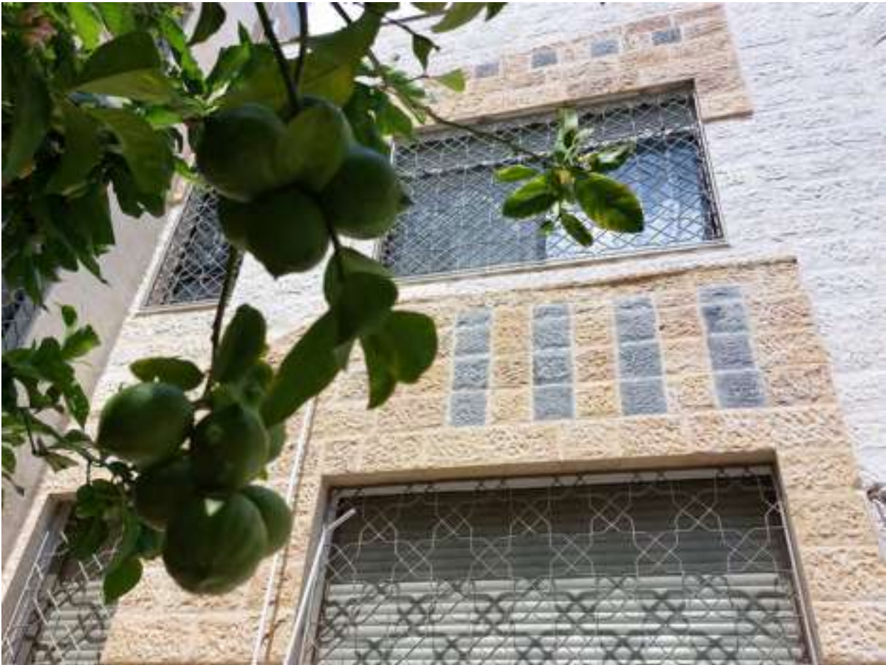
Figure 12 Side Facade with Stone Window Framing. Safadi Villa- Irbid, Jordan.
