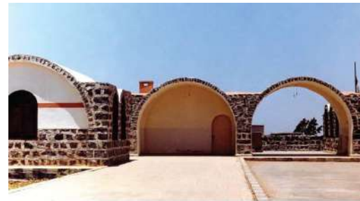
Classroom block with archway, rear view
