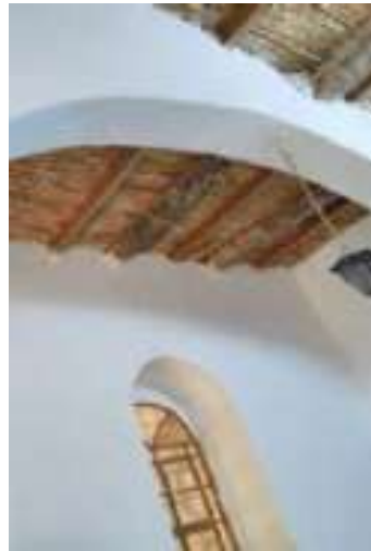
9- The wooden trunk and reeds roofing system using arching support construction in Arar's house
