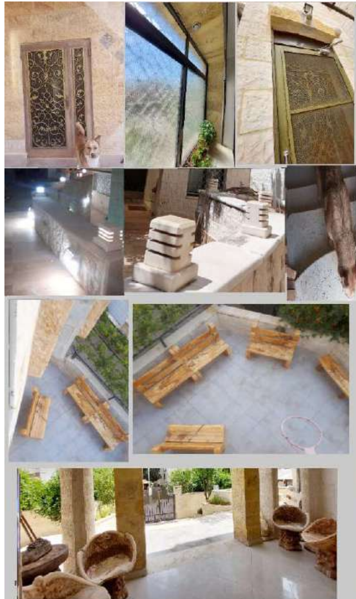
Figure 18 Interior- Exterior Finishing. Safadi Villa- Irbid, Jordan.
