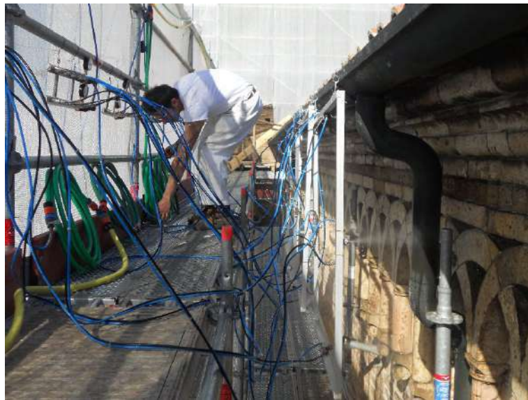
1 Cleaning with demineralized water system
