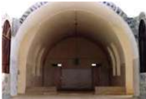
Archway leading to administration rooms
