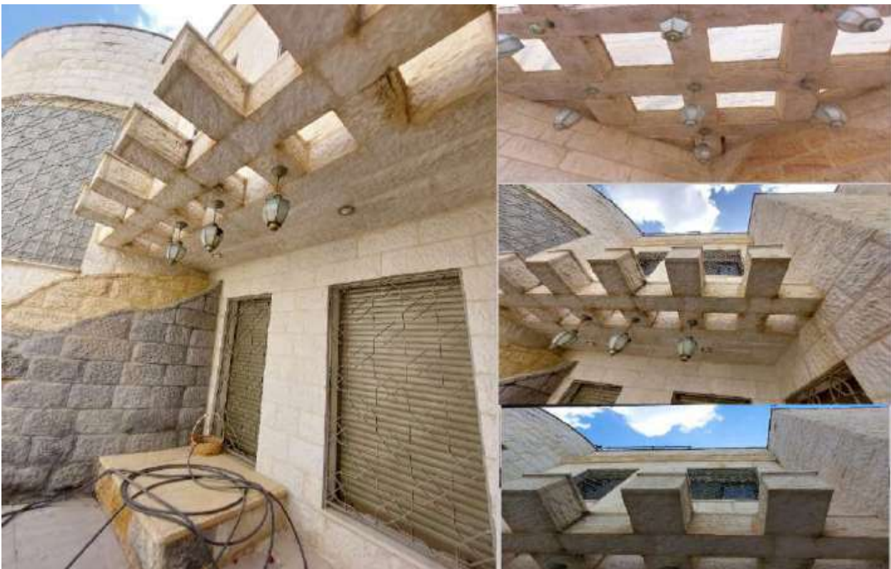
Figure 9 Exterior Lighting. Safadi Villa- Irbid, Jordan.
