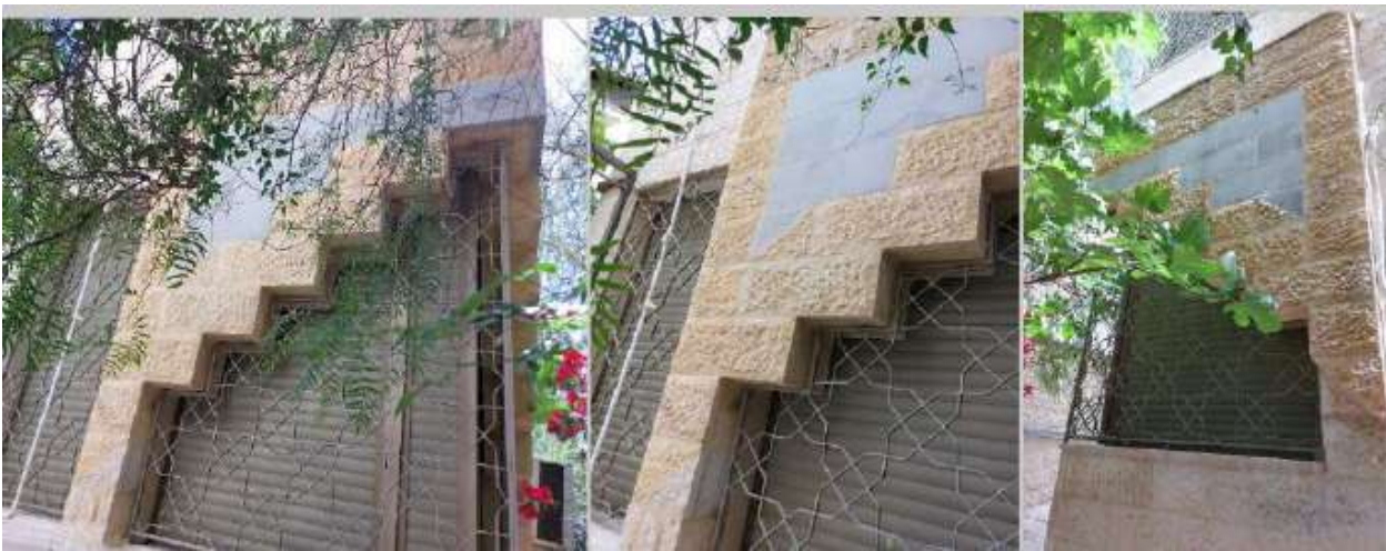
Figure 8 Window Arches and Frames Made from Three Different Stone Types. Safadi Villa- Irbid, Jordan.
