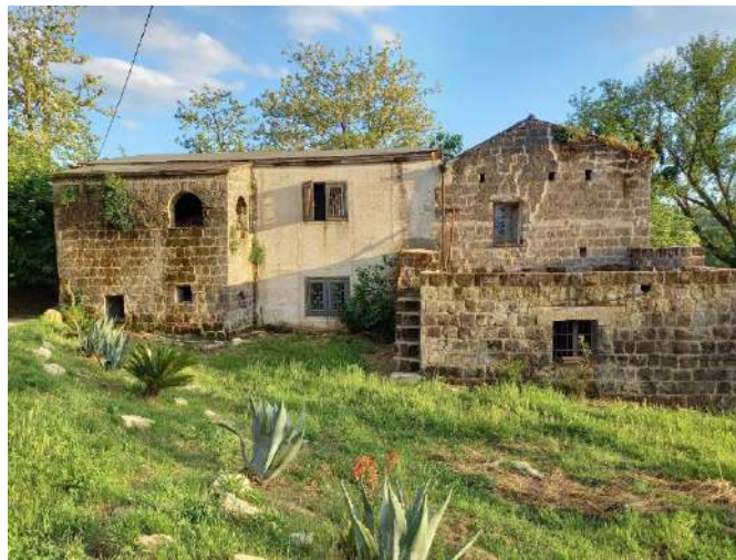
8 – post-renovation north facade.
