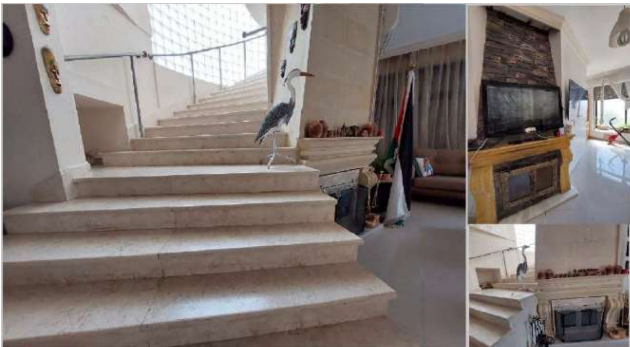
Figure 17 Interior Use of Stone- Finishing: Stone Fireplace and Stone Stairs. Safadi Villa- Irbid, Jordan.
