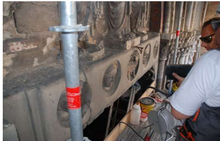
4 Stone cleaning with laser
