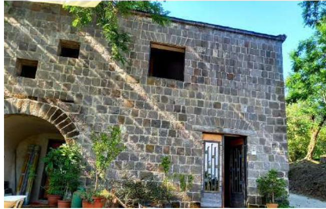
7 – post-renovation south facade.
