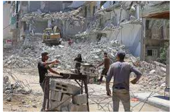
6. Gazan worker recycle rubble as Israel upholds ban on construction goods . Source: Al Jazeera, 17 Jun 2021
