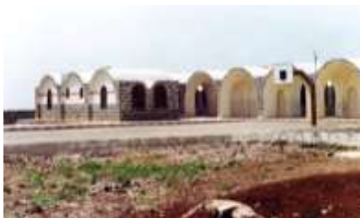
view from the south with administration to the left
