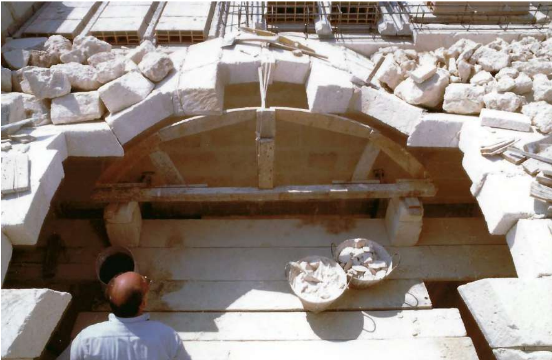
Photo 6: the four groin sections are almost complete, and now the sail vault portion will be constructed.
