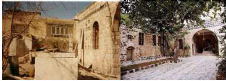
3- Arar's house before and after restoration
