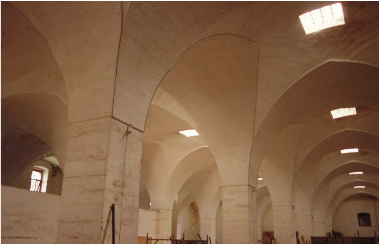
Photo 9: example of a building covered with large spigolo vaults, without the keystone closure.
