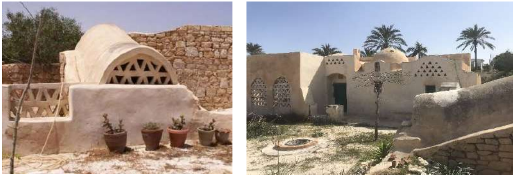
Fig 2: Artesian Well vault
