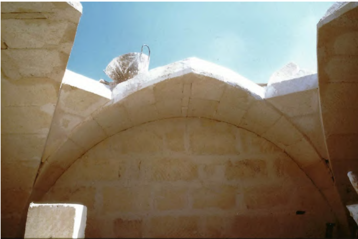
Photo 7: Groin sections completed. Final stage of the vault construction.
