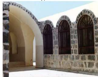
Close-up showing exposed stonework on facade
