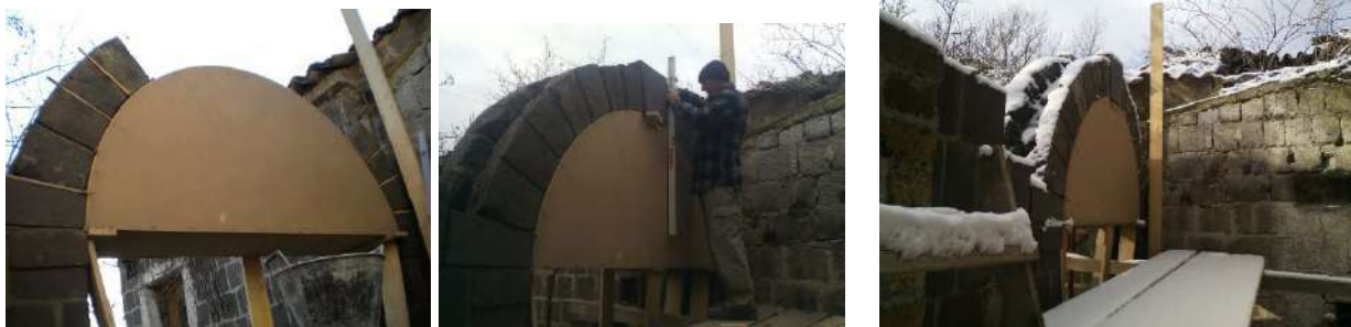
6 – the gray tuff arch in its construction phases - south facade.
