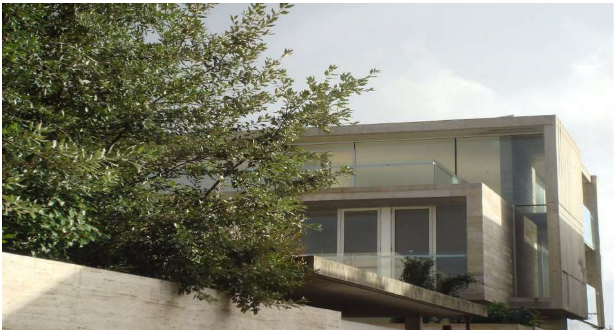
6 – Terraced Houses, San Marcellino, Italy
