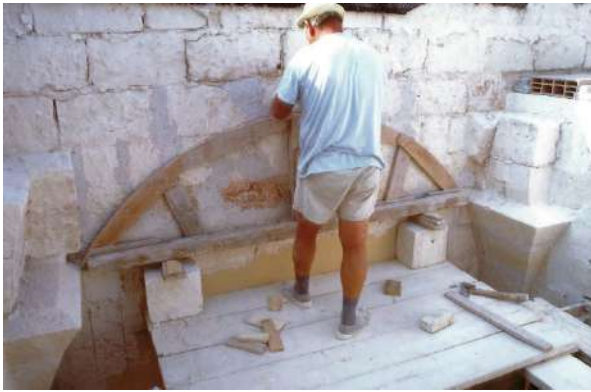
Photo 3: the worker positions the forma volante on the wall to trace the arch of the vault.
