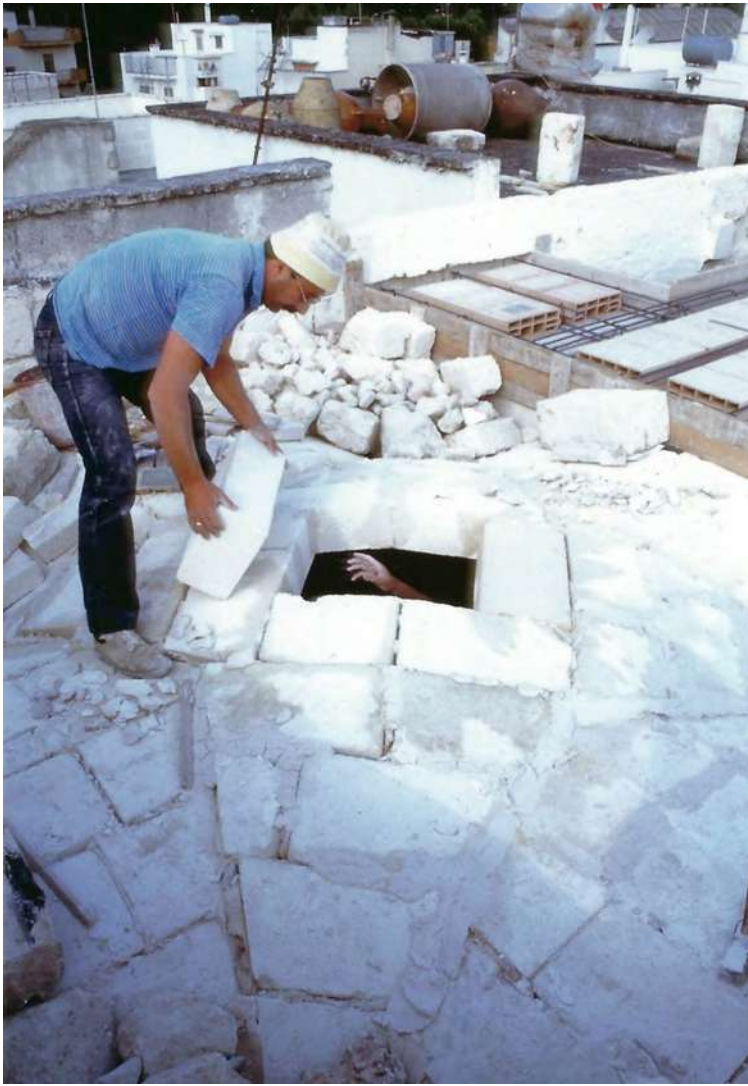
Photo 8: the closing stage of the vault, called toppa (keystone).
