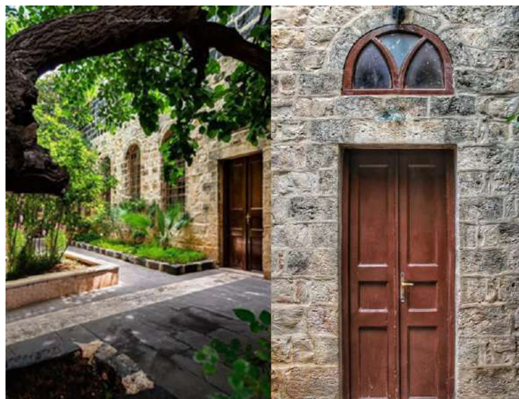
10- Wood was used in both doors and windows
