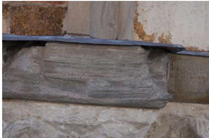
5 Grouting surface cracks with lime mortar
