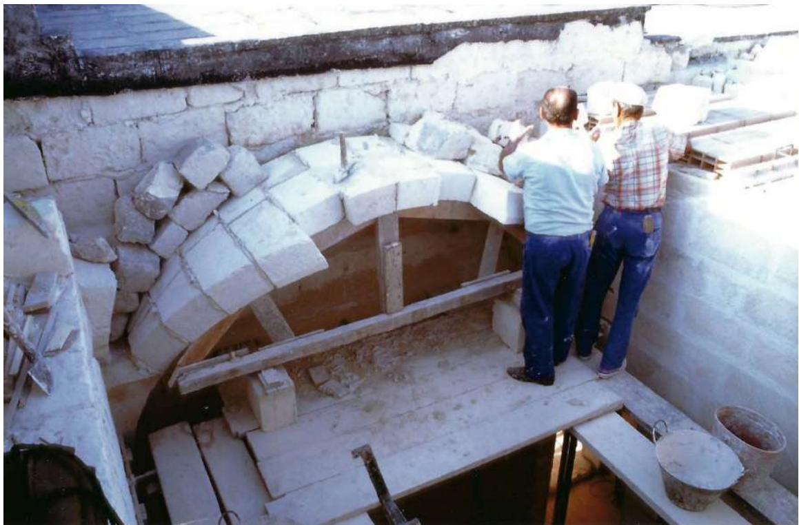
Photo 5: the forma is progressively moved forward as the groin section progresses. At the same time, the side walls are loaded.
