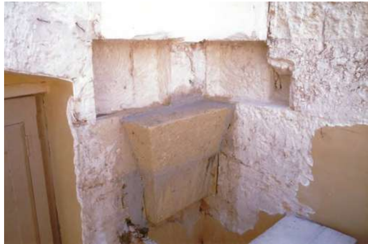
Photo 2: the blocks of the appese are positioned in the corners of the wall.
